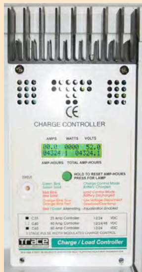
Figure 73. Charge controllers used in PV systems vary widely in their size, functions and features.
