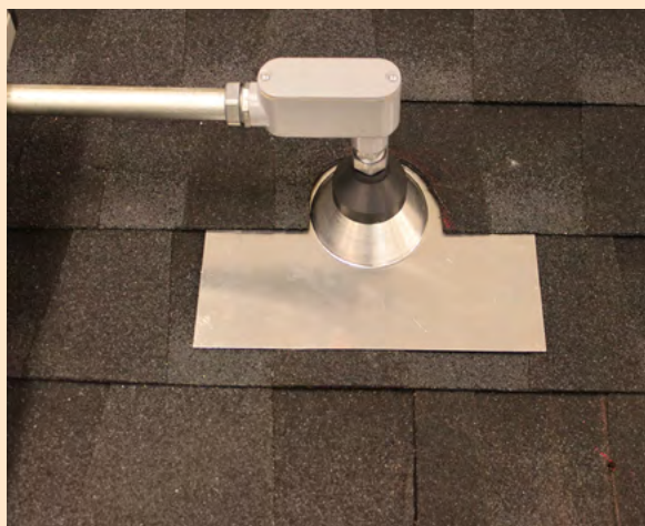
Figure 96. Flashed conduit penetration
