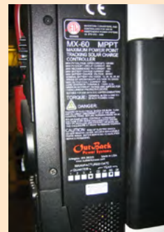
Figure 73. Charge controllers used in PV systems vary widely in their size, functions and features.
