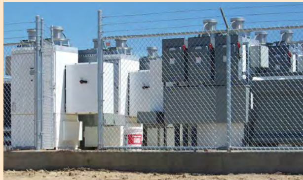
Figure 57. Utility-scale inverters use higher DC input and AC output voltages to reduce losses, and the size and costs of the conductors and switchgear required.
