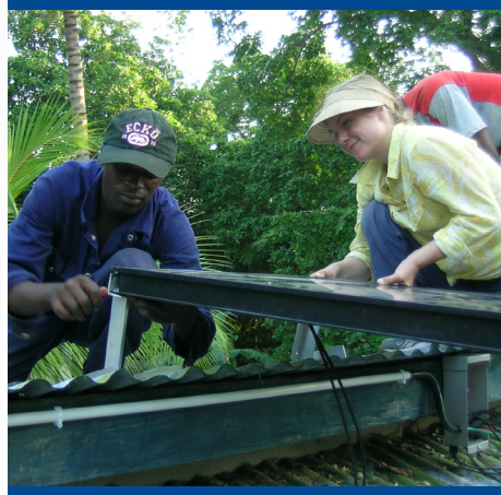
Goldah volunteering, in Tanzania, to install PV panels on a community learning center.
