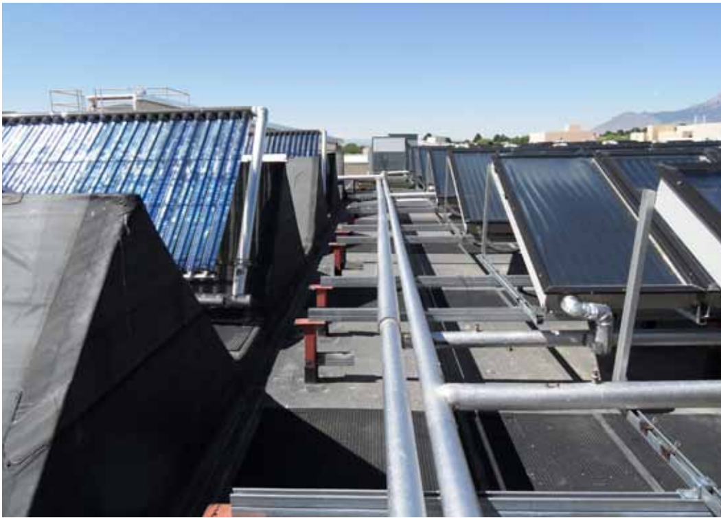
Figure 8-56 — Aluminum cladding used to protect pipe insulation from UV-degradation
