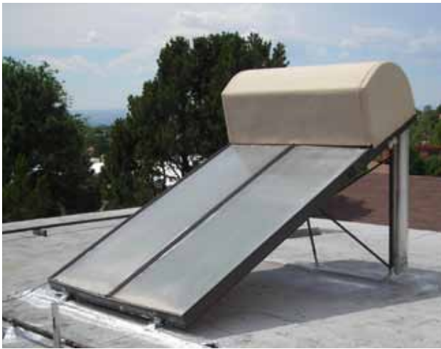
Figure 4-17 – Indirect Thermosyphon System.
