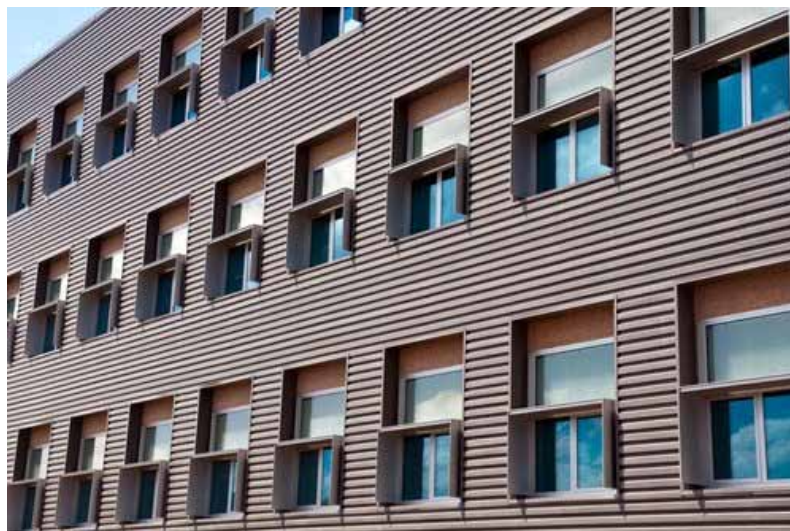
Figure 4-11 — Transpired solar air collectors are similar in appearance to corrugated metal siding. This installation utilizes nearly the entire available wall area for solar collection. (Courtesy of the National Renewable Energy Laboratory)
