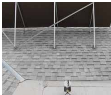
Figure 8-10 – Climate plays a significant role in the suitability of materials. The image on the left is a painted steel rack supporting aluminum-framed collectors in the southwestern United States. After ten years there is no sign of corrosion. A similar installation in the northeastern U.S. creates significant galvanic corrosion between dissimilar metals, as can be seen on the right. (Courtesy of NYSERDA)
