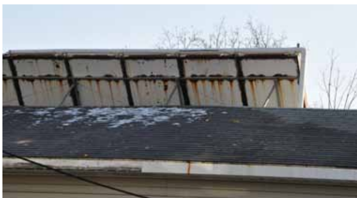
Figure 8-10 – Climate plays a significant role in the suitability of materials. The image on the left is a painted steel rack supporting aluminum-framed collectors in the southwestern United States. After ten years there is no sign of corrosion. A similar installation in the northeastern U.S. creates significant galvanic corrosion between dissimilar metals, as can be seen on the right. (Courtesy of NYSERDA)
