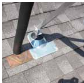
Figure 8-30 — Flashing of pipe penetration and cylindrical standoff. (Courtesy of Liquid Solar Systems)
