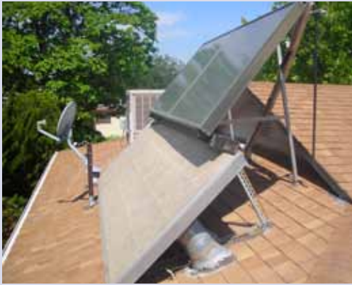
Figure 10-38 — Stacking collectors with wood mounts?
