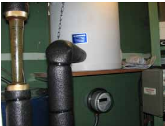
Figure 10-5 — The flow meter on the left can be used as a sight glass in a drainback system when placed at the proper level.
