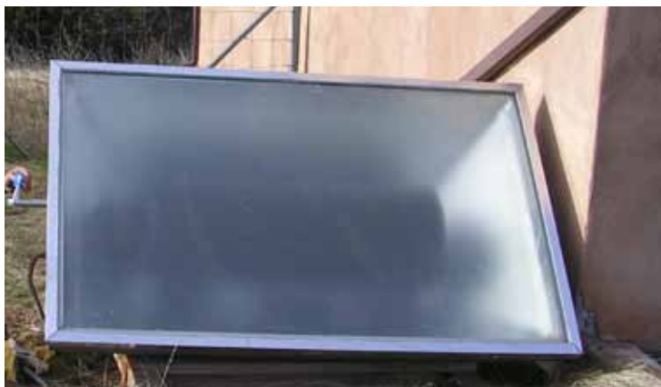
Figure 10-1— Batch solar water heater.
