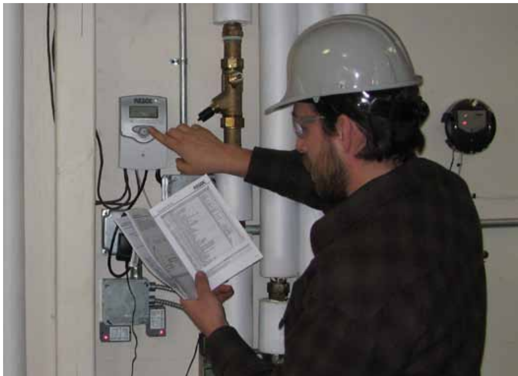
Figure 9-1 — Programming a differential controller.
