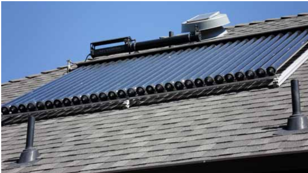
Figure 10-22 — Overflow reservoir used as a heat dump above an evacuated tube collector.
