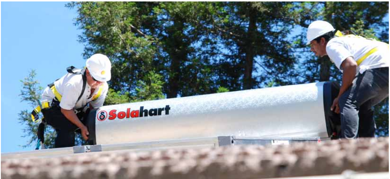
Figure 8-18 — Installation of an ICS thermosyphon system.
