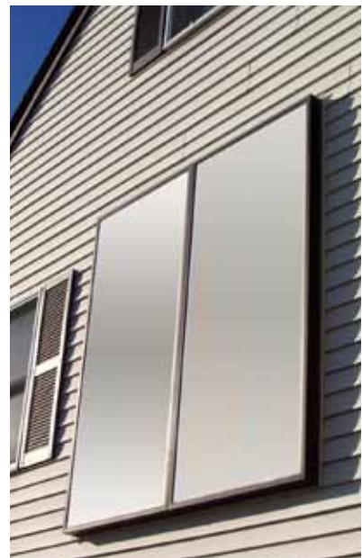
Figure 4-9 — Glazed solar air heater. (Courtesy of Environmental Solar Systems)
