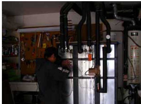
Figure 10-29a and b — Internal view of a bladder tank with heat exchangers and external view of a similar tank installed in a garage. The unpressurized atmospheric tanks are the least expensive method of storing large quantities (hundreds of gallons) of hot water for commercial systems or home space heating.
