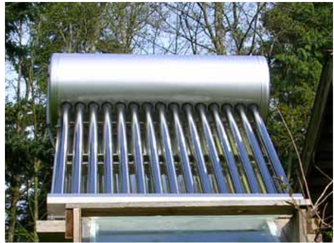
Figure 4-18 – Unpressurized Thermosyphon evacuated tube system.
