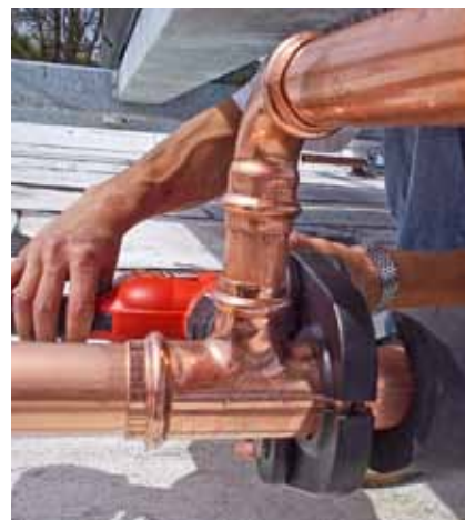
Figure 8-36 — Pressing tool used to crimp specialized fitting; the raised ring on the fitting houses an o-ring that seals between the fitting and the tubing.
