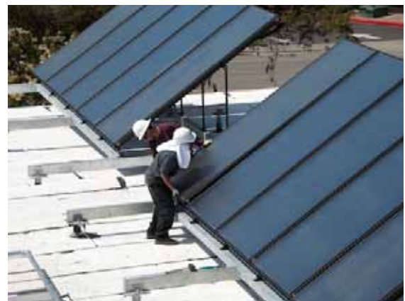
Figure 10-23 — Large systems may require that collector arrays are plumbed in multiple banks to limit frictional head loss.
