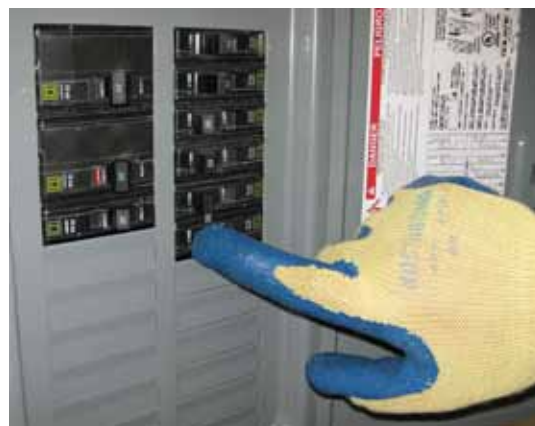
Figure 10-2— The hot water heater breaker at the electrical panel must be shut off prior to any service work. Energizing a water heating element that is not submersed in water will immediately damage it.
