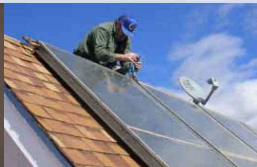
Figure 10-45 — Maybe too steep without fall protection?
