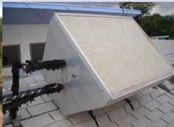
Figure 10-37 — Insulation doesn't stay on piping without protection; will the collector stay on the roof?
