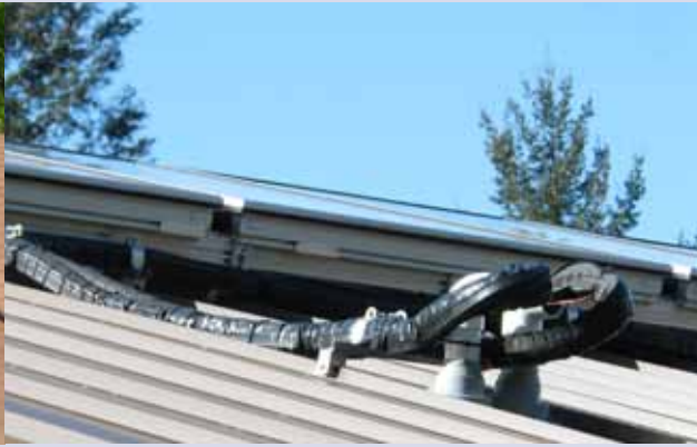
Figure 10-39 — Pipe snake—what problems could this detail cause?
