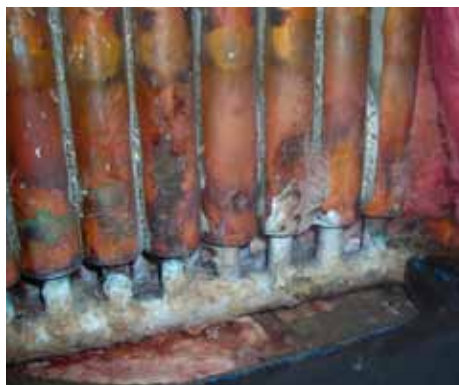
Figure 10-26 – Corrosion in a copper tube heat exchanger.
