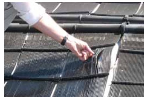
Figure 10-11 — Leaking pool collector (note the water on the riser tubes).
