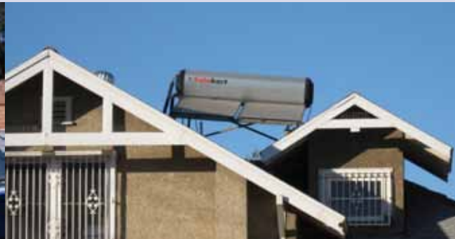
Figure 10-35 — Self-leveling ICS system.
