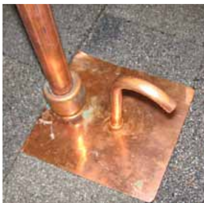
Figure 8-31 — Copper pipe flashing with gooseneck for sensor wire. A collar is soldered to the copper plate flashing and concealed under the copper cap in this photo. The copper cap is soldered to the copper tubing. There is no connection between the collar and the cap or the collar and the piping; this allows the tubing to expand and contract without affecting the integrity of the copper flashing plate.
