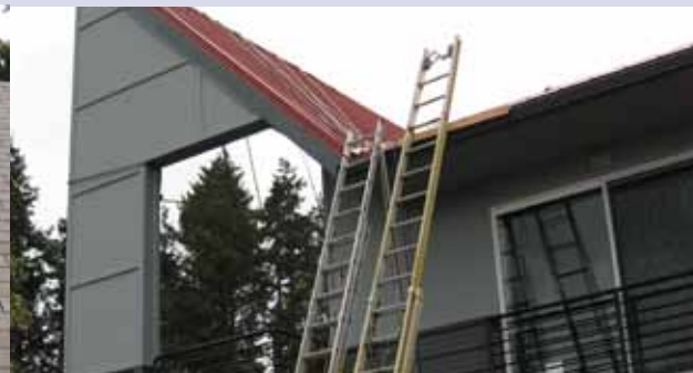
Figure 10-43 — Know your ladder set up rules
