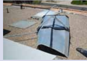
Figure 10-31 — Poorly secured collectors are victims of the wind.
