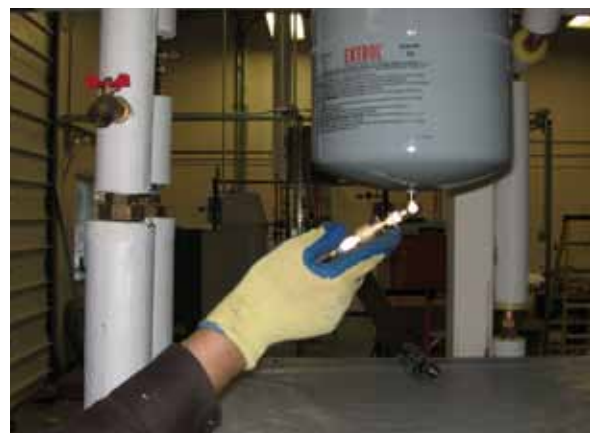
Figure 8-49 – Pressurizing an expansion tank with compressed air.
