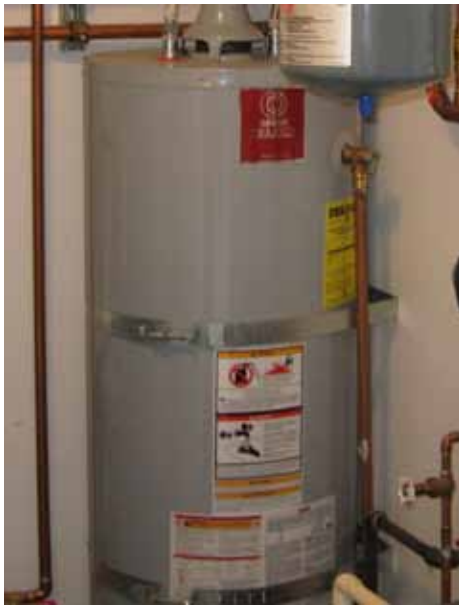
Figure 8-45 — Earthquake strap for a standard water heater.
