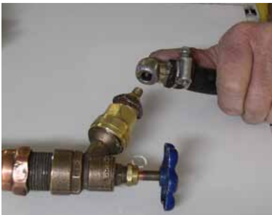
Figure 8-37 – Filling the system with compressed air.
