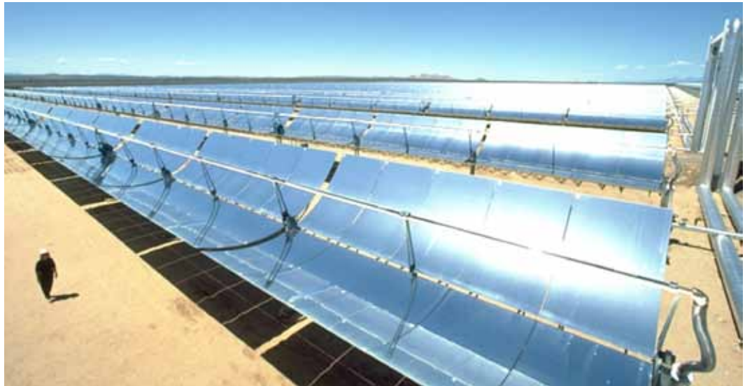
Figure 4-12 – Parabolic trough collectors at Kramer Junction, CA. (Courtesy of Sandia National Laboratories, photo credit Greg Kolb)
