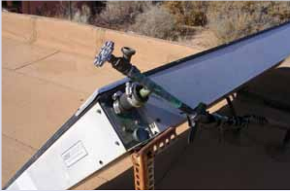
Figure 10-32 — Antifreeze system — roof work.
