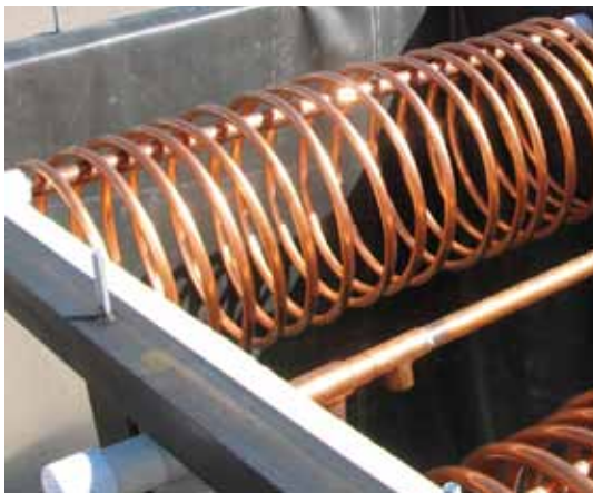
Figure 10-29a and b — Internal view of a bladder tank with heat exchangers and external view of a similar tank installed in a garage. The unpressurized atmospheric tanks are the least expensive method of storing large quantities (hundreds of gallons) of hot water for commercial systems or home space heating.
