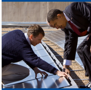
Blake Jones of Namaste Solar shows President Barack Obama and Vice President Joe Biden the ballast trays of a T-10 flat roof mounting system on top of the Denver Museum of Nature & Science, February 2009.
