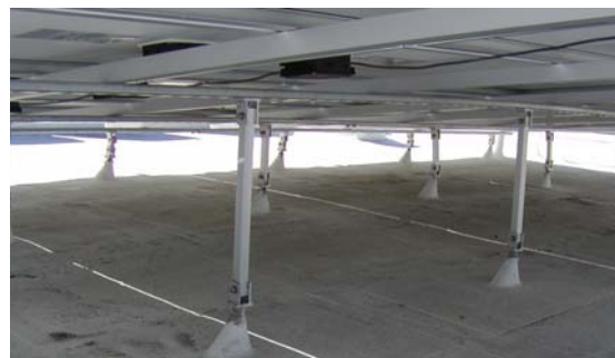
Figure 9 Flashed Penetration (correct)
