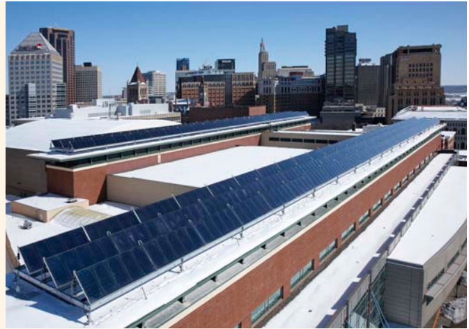
Figure 6-12 — View of collector array for the solar thermal District Energy project. (Courtesy of District Energy St. Paul)
