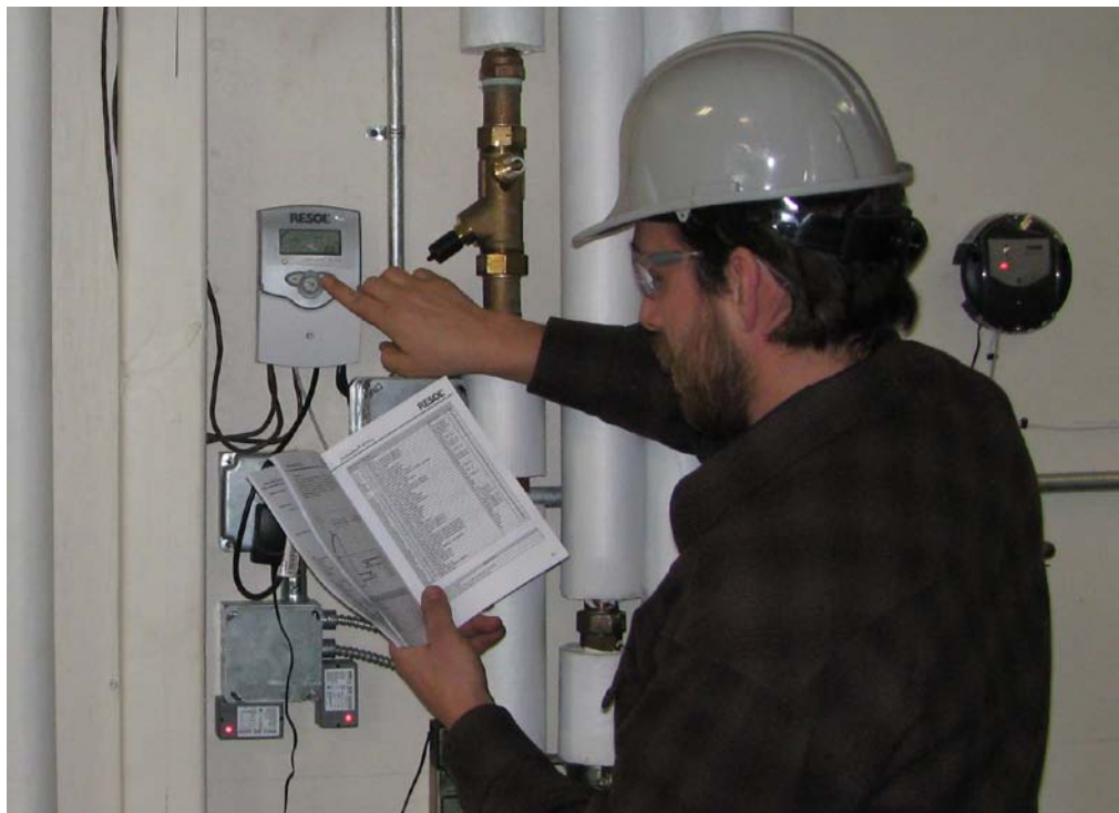
Figure 9-1 — Programming a differential controller.
