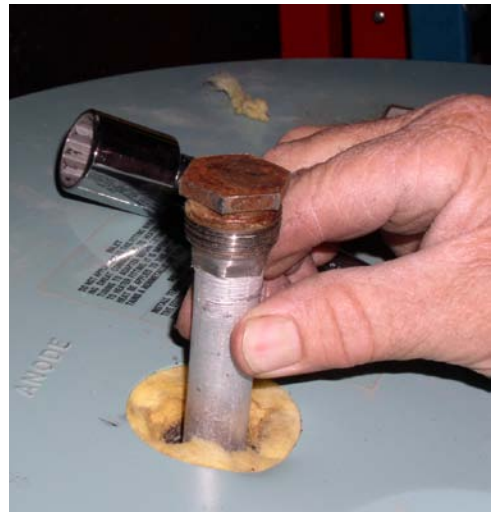
Figure 10-9 — The anode rod may have a separate port on the top of the tank.
