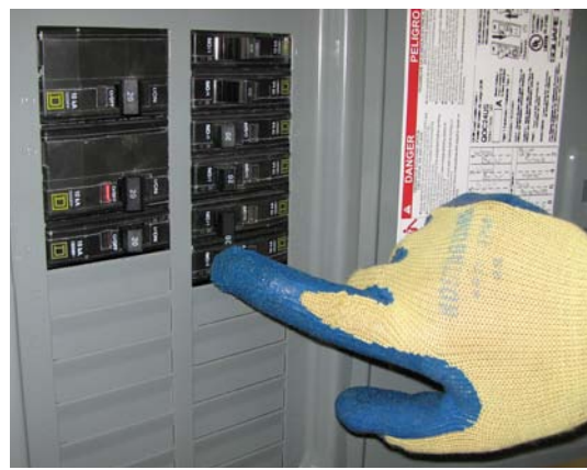
Figure 10-2— The hot water heater breaker at the electrical panel must be shut off prior to any service work. Energizing a water heating element that is not submersed in water will immediately damage it.
