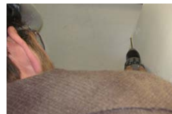
Figure 7-1 – Drilling a pilot hole from below to locate roof rafters.
