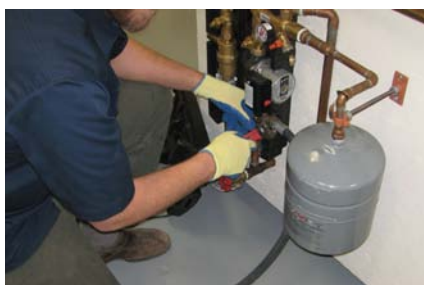
Figure 8-55 — Connecting a glycol filling station to the pump station fill valve.
