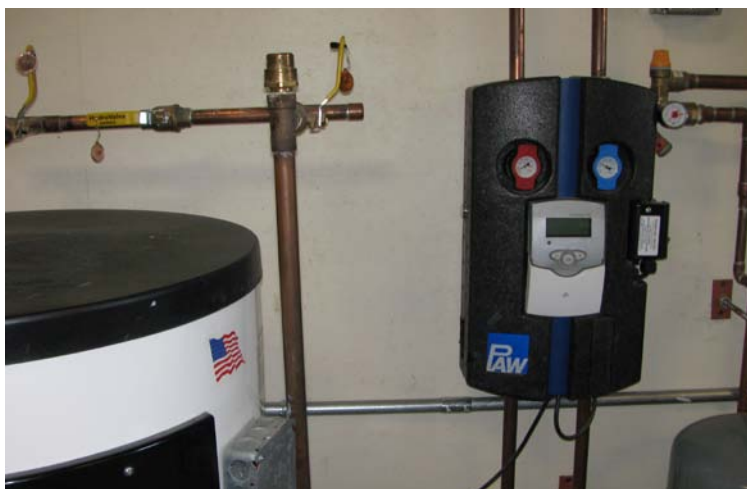
Figure 7-3 — It is often beneficial to locate the pump station and controls near the storage tank.
