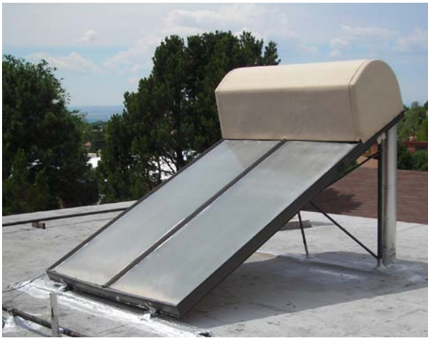
Figure 4-17 — Indirect Thermosyphon System.
