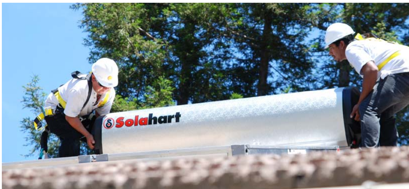
Figure 8-18 — Installation of an ICS thermosyphon system.
