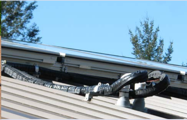
Figure 10-39 — Pipe snake—what problems could this detail cause?
