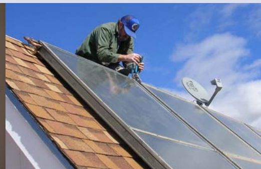
Figure 10-45 — Maybe too steep without fall protection?
