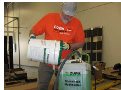
Figure 8-54 — Filling the charging station with a solution of propylene glycol and water.
