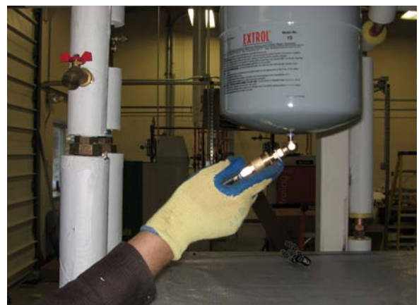
Figure 8-49 – Pressurizing an expansion tank with compressed air.
