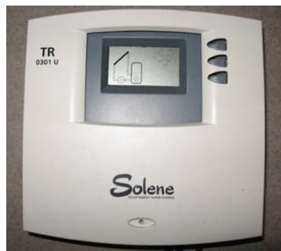
Figure 10-21 — Differential controllers can also be used to dissipate heat at night by turning on the system pump when the tank is too hot. This feature is called vacation mode in some controls.
