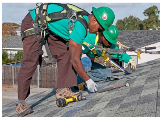
Figure 8-3 — Solar installers wearing proper fall protection, including safety harnesses, lanyards, rope grabs, and safety ropes. (Courtesy of Shawn Schreiner)
