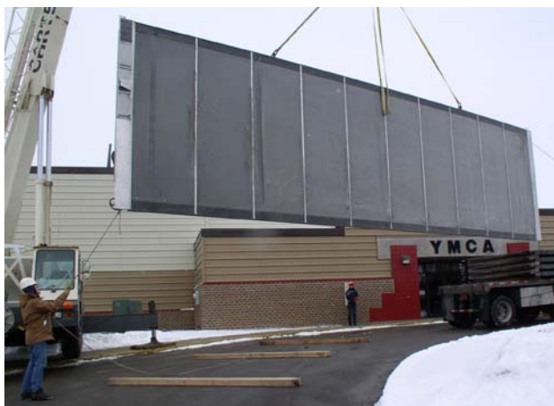
Figure 8-17 — Using a crane to transport pre-mounted collectors to the roof.
