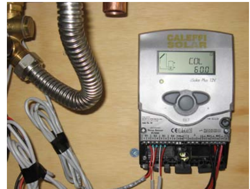
Figure 10-17 — A differential controller with the face removed to check sensor and pump wiring.
