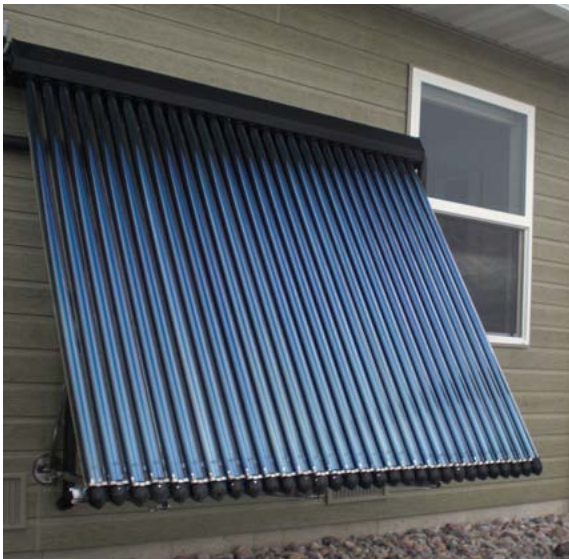
Figure 8-13 — Wall-mounted evacuated tube collector. (Courtesy of Liquid Solar Systems)
