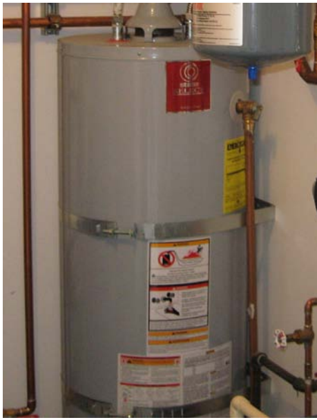
Figure 8-45 — Earthquake strap for a standard water heater.
