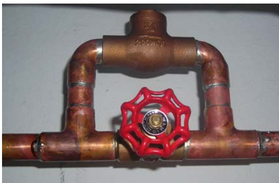
Figure 10-20 — Check valve bypass for nighttime cooling. Under normal operation the gate valve in this photo is closed. When opened, the valve allows reverse flow by thermosyphoning. Heat can be re-radiated to the colder sky if flat plate collectors are utilized.
