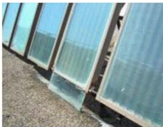
Figure 10-12 – This collector's frame is no longer holding the glazing in place and needs repair.
