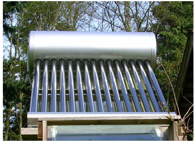
Figure 4-18 — Unpressurized Thermosyphon evacuated tube system.
